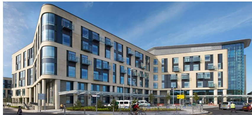
Maintenance at Southmead Hospital – United Kingdom – €159m
