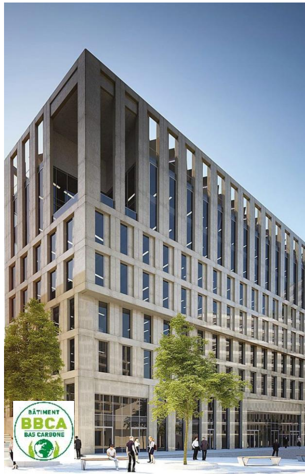
Bouygues Immobilier was awarded the BBKA (low-carbon building) label for Enjoy, the largest timber positive-energy office building in France
