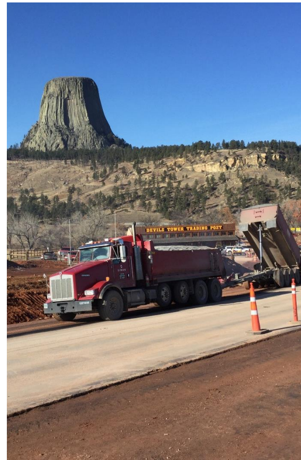
Roadworks at Devils Tower in Wyoming – USA
